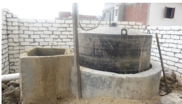
Fig. (1): A photo of the digester and gas holder
