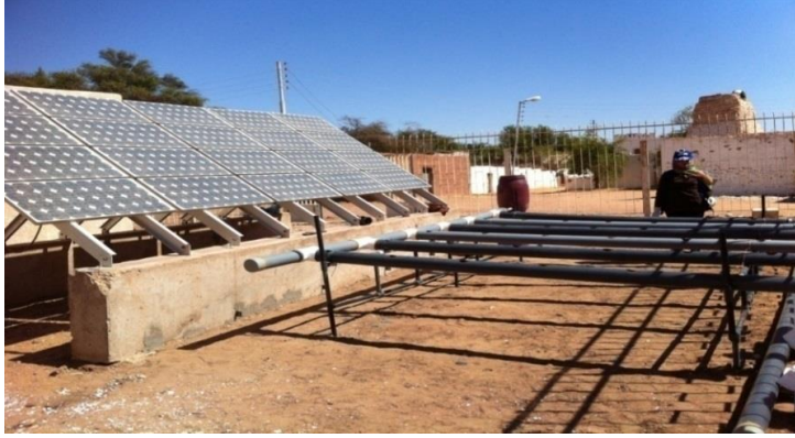
Fig.(1):System including solar pump and hydroponic unit.
