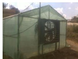
b- Mechanically ventilated greenhouse (GH2)
