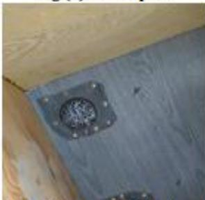
Fig.(7)Two screened bottom holes
