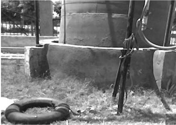
Figure (2): biogas filling system from gas holder to inner tube
