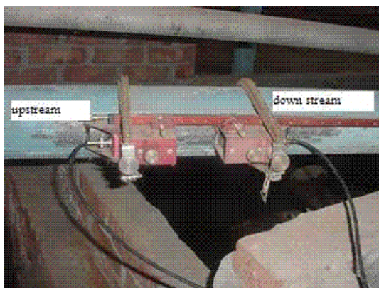
Figure (11): Mounting U-S. flowmeter on steel pipe.
