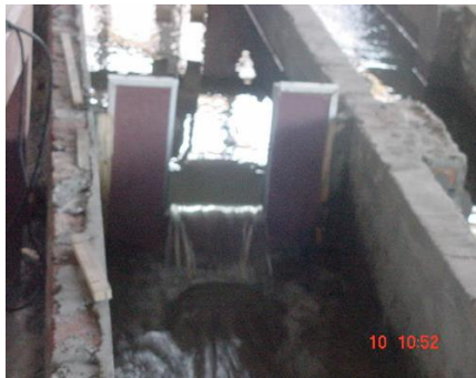
Figure (4): Rectangular weir.
